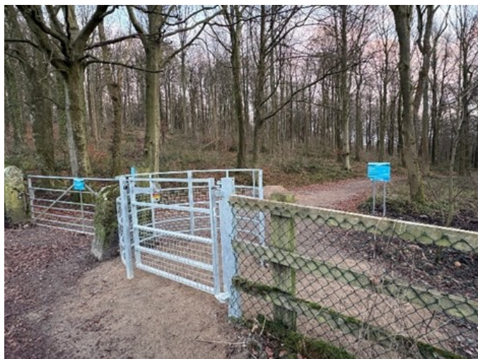
Gaps are ideal, but this RADAR kissing gate replaced a very rickety stone stile at Fewston
